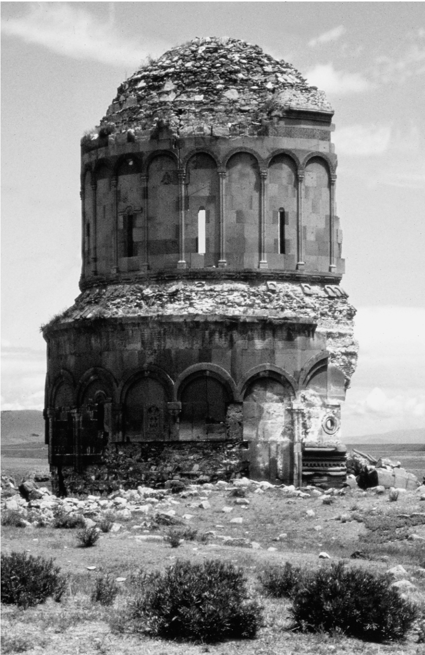
5.3 South façade, Church of the Holy Saviour, Ani
